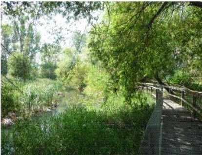
Extensive environmental restoration, especially when incorporated as an amenity as in this case
