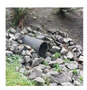
Example of energy dissipation to prevent erosion. This technique is used for both construction and permanent stormwater controls
