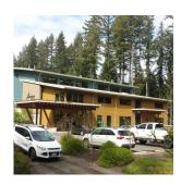
The City's maintenance and operations center incorporated many LID features including a green roof (above) and infiltration pond (below)
