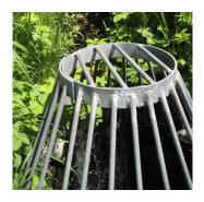
Example birdcage structure used to prevent large debris from getting into and clogging stormwater pipes. City crews inspect and maintain these facilities
