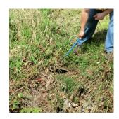
Roadside ditch in need of maintenance. Vegetation is blocking inlet to pipe.
