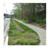
Example of curb cuts and porous concrete stormwater retrofit on 233rd Avenue NE
