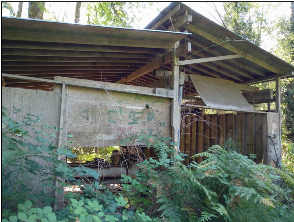
Figure 12. View of the outbuilding (age unknown); view is to the southwest.
