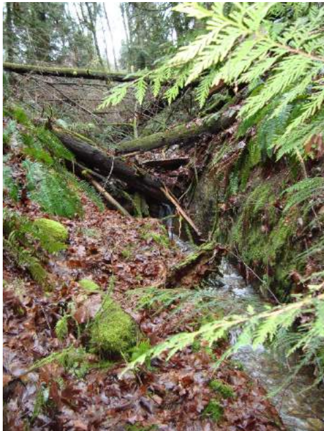
Site location: ~1,275' upstream of 206 th Avenue NE Photo number: Z-30 Description: Looking upstream at debris jam in channel. Lots of downed trees and narrow channel through this reach.
