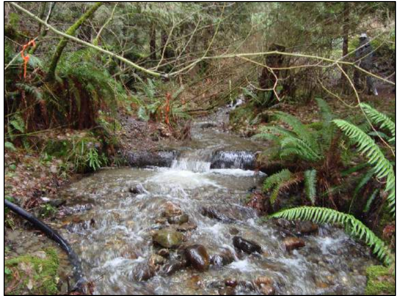
Photo 5- 5. Log grade control structure in channel downstream of confluence with south tributary. Pipe shown on the left of photo is water intake for salmon incubation boxes. January 12, 2018.
