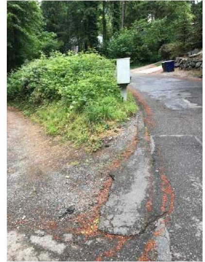
Intersection of 210th Ave NE and Louis Thompson Rd. (right photo)
