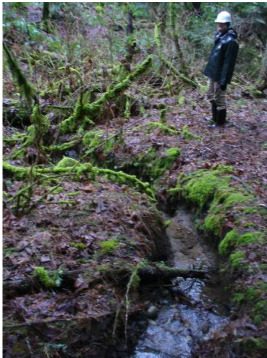
Site location: 150' upstream of birdcage east of 206 th Ave NE Photo number: Z-46 Description: Deeper incision in the upstream direction.
