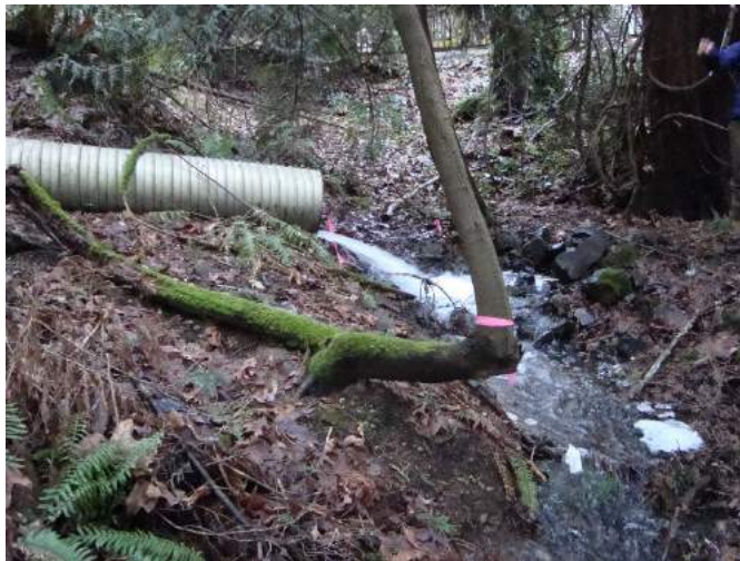
Site location: ~2,100' upstream of 206 th Avenue NE Photo number: Z-40 Description: Looking upstream at culvert (Outfall 5) discharging water to form the headwaters of Zackuse Creek.
