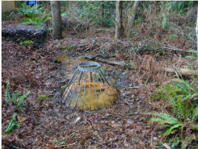
Site location: ~ 1100' upstream of birdcage east of 206 th Ave NE Photo number: Z-55 Description: Looking downstream (west) at birdcage outfall and gabion structures behind it. Location is near SE 3 rd Street. Headwaters of S. Tributary.
