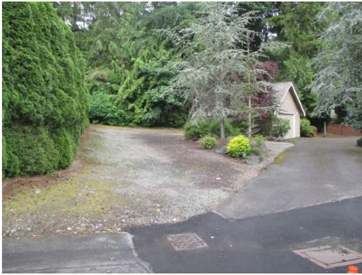
East Montage vault (under gravel drive) and catch basins (foreground)
