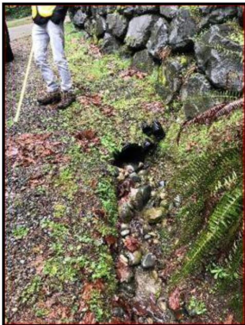
Louis Thompson Road culvert. April 2018.
