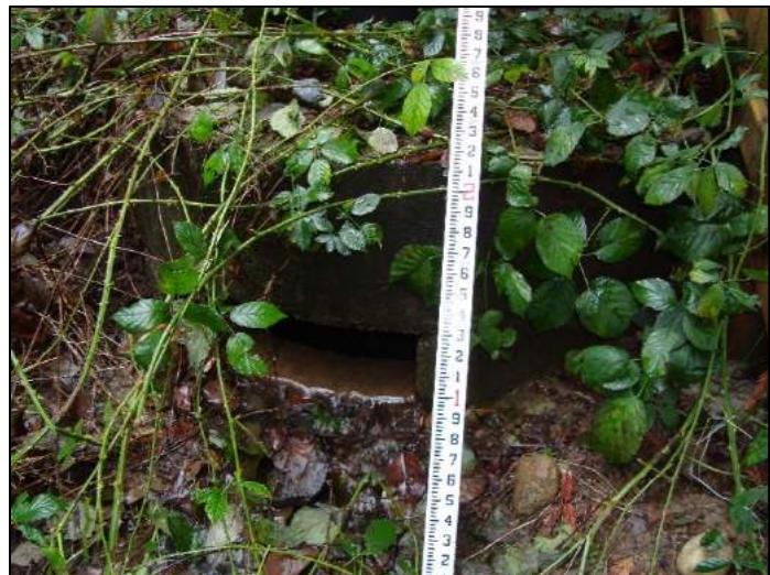
Photo 5-12. Tamarack outlet structure at top of Tamarack Ravine. January 12, 2018.
