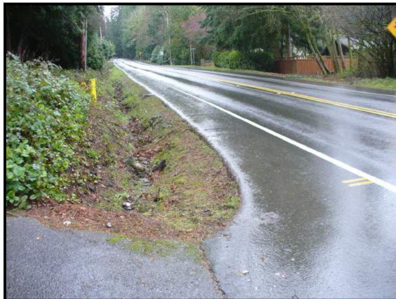
Louis Thompson Road ditch. March 2018.
