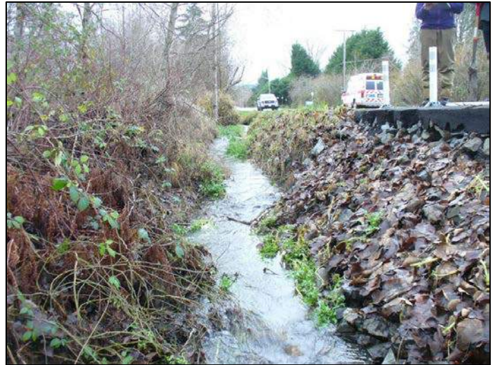
Photo 5-17. Zackuse Creek flowing in ditch along E Lake Sammamish Parkway prior to late summer 2018, when the creek was realigned away from the road. Photo is looking to the south. January 12, 2018.
