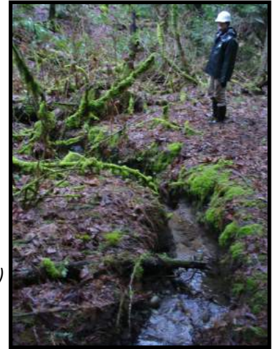
Stream channel erosion (right photo)
