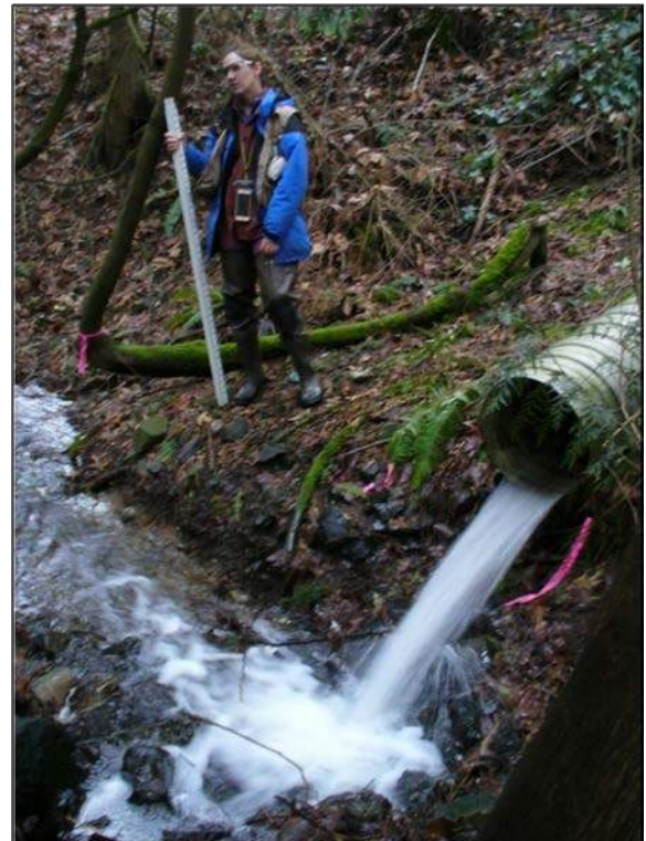
Photo 5-1. Headwaters of Zackuse Creek. Creek flow originates in 18-inch-diameter pipe, as shown above. Photo taken looking north on January 12, 2018.
