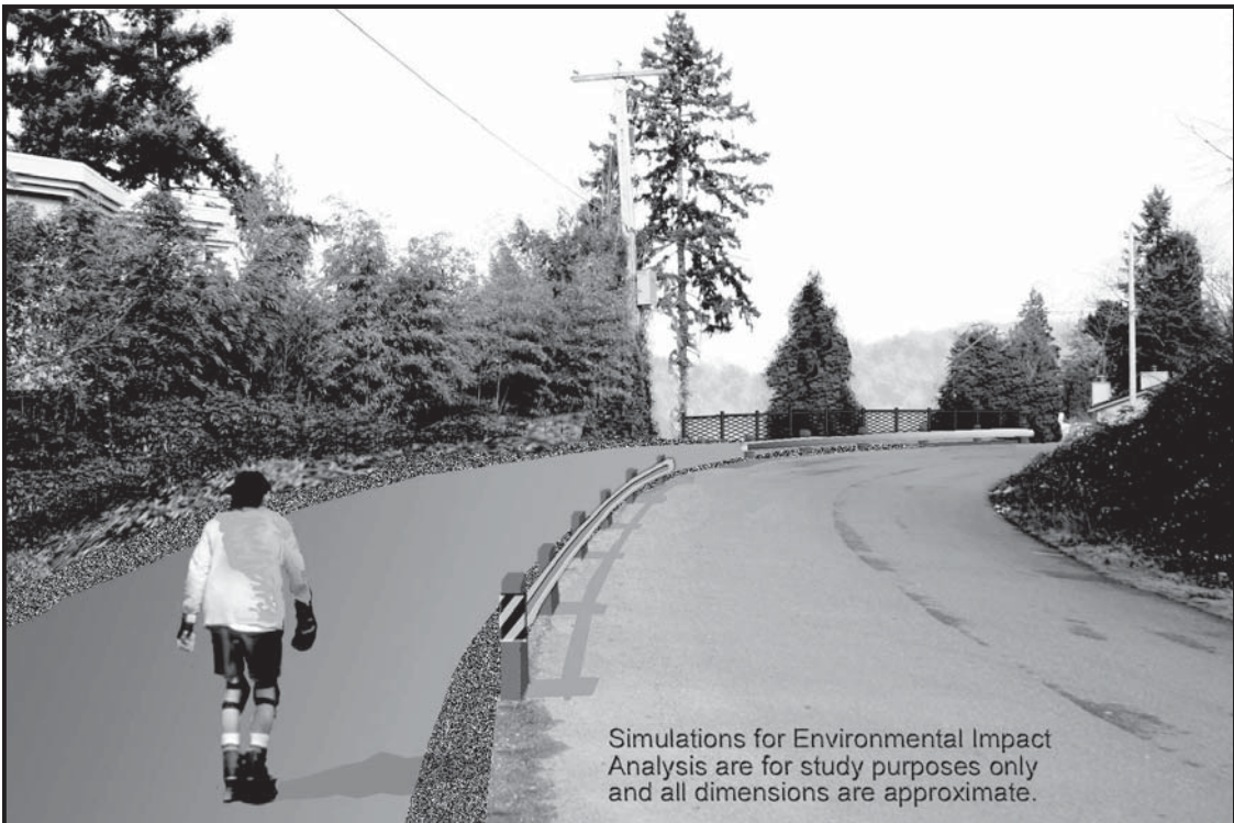
East Alternative; Looking north from about 2100 block on E Lake Sammamish Place SE. Paved path is 12 ft. wide with 2 ft. shoulders.
