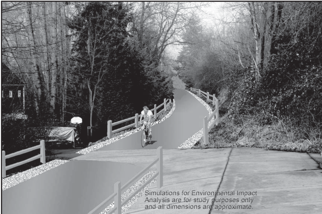
Corridor Alternative; Looking northwest from railbed and driveway across from NE 33rd Place. Paved path is 12 ft. wide with 2 ft. gravel shoulders.
