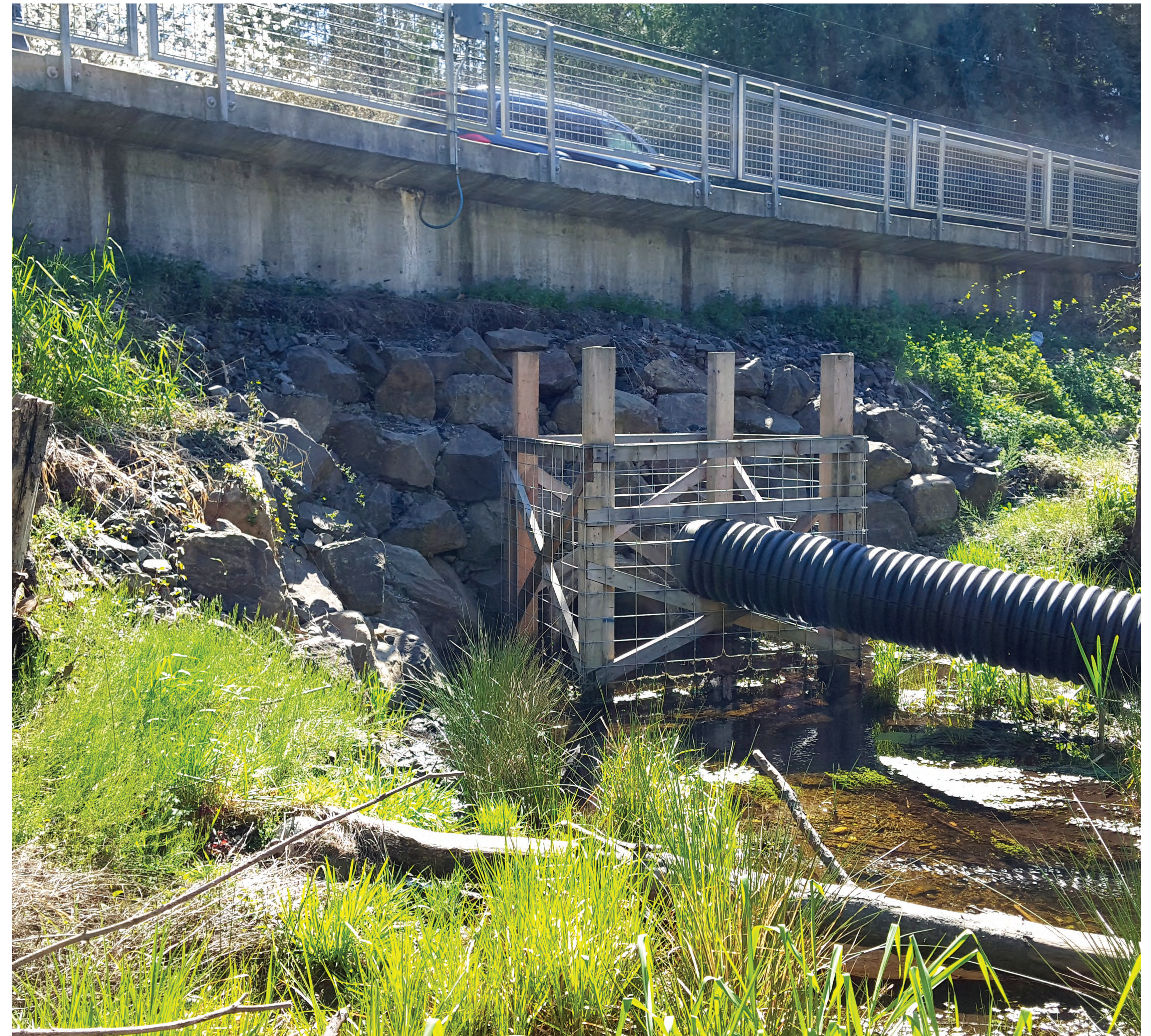
Current North Fork Issaquah Creek Culvert
