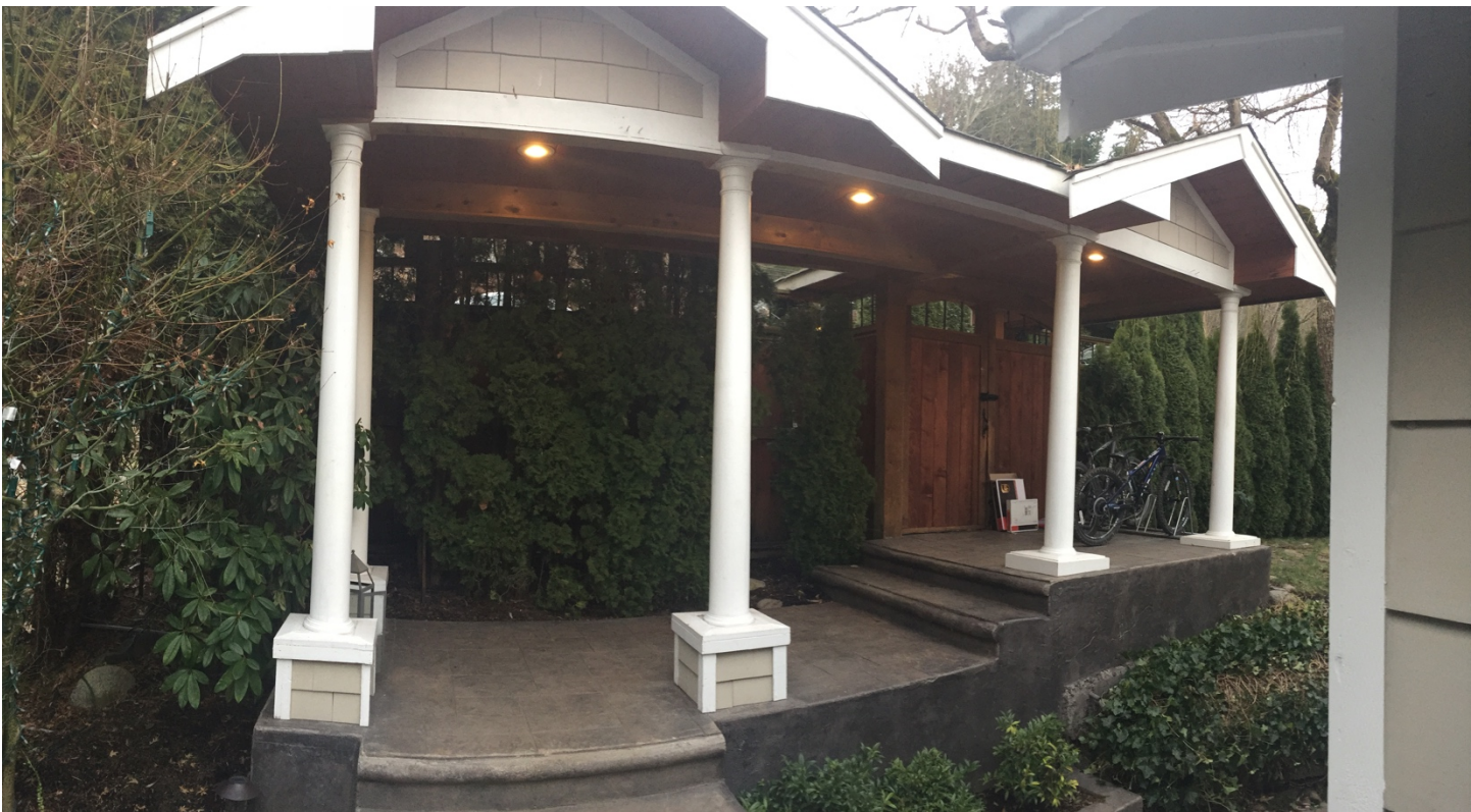
Elevation doesn't match up with 60% plan. Needs to be restored
